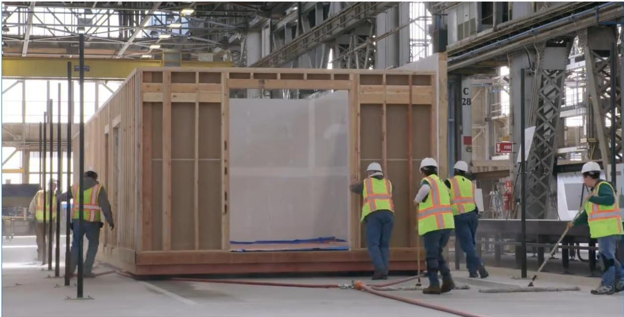
*Positioning a large structure in a precise location is more ergonomic and reliable when it is floating on air instead of using a forklift, crane, or rail system.*
