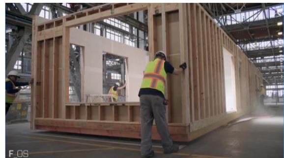
*It takes less than 10 minutes to lift and move a 50' long, 30,000 lb. structure from workstation to workstation using air bearings.*
